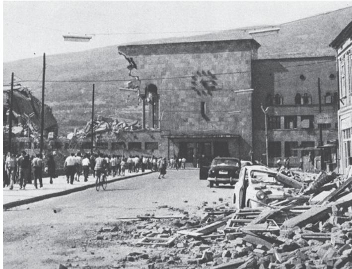
Figure 1. The Railway Station (now City Museum) after the earthquake in 1963
