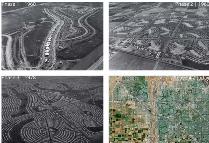
Figure 2. Sun City's the different phases of construction.
