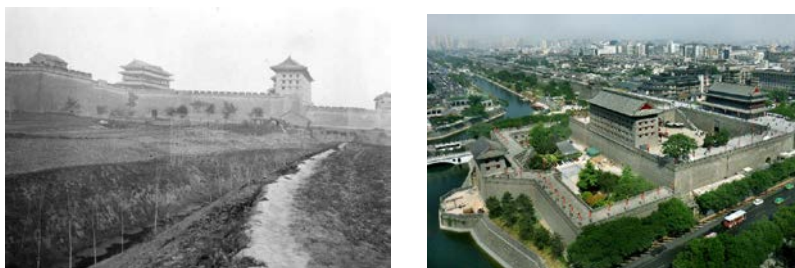
Figure 5. Xi'an, south gate section of city wall, previous state in 1912 and present state in 2014
